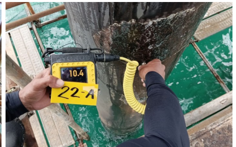
Ultrasonic Thickness Gauge (UTG) Test
