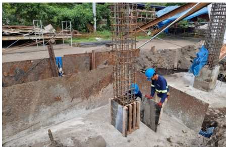
Construction of Hangar 1
