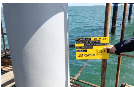
Application of Paint
