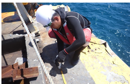
Rebound Hammer Test
