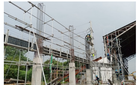
Construction of Hangar 1
