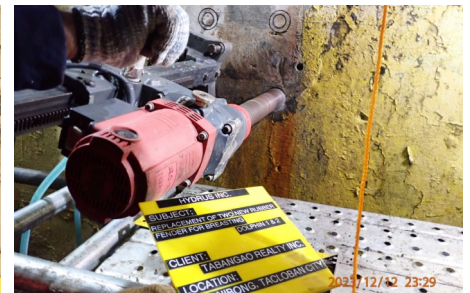
Coring of New Holes for Fender
