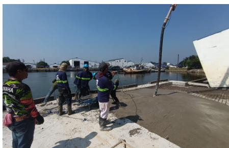
Construction of Wharf
