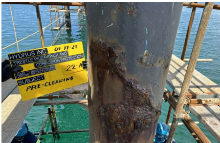
Pre-cleaning of Corroded Steel Pipe Piles
