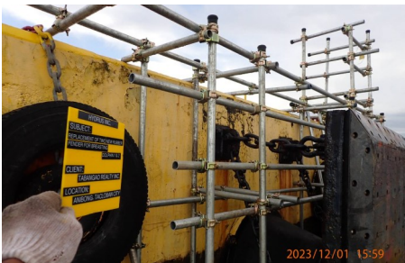
Erection of Scaffolding
