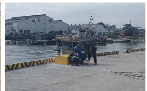
Installation of Shore Power
