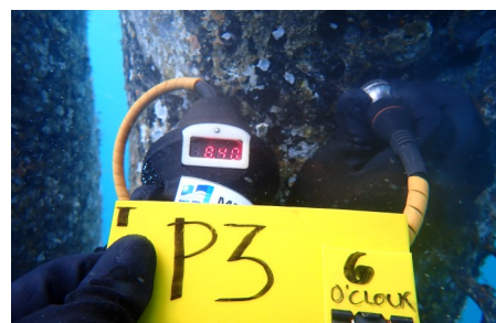
Ultrasonic Thickness Gauge (UTG) Test
