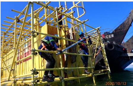
Erection of Scaffolding
