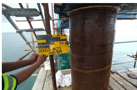
Application of Petrolatum Paste and Tape
