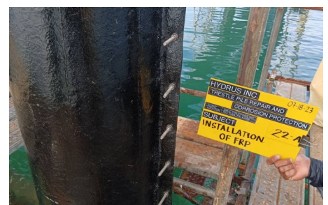
Encapsulation of Fiber-Reinforced Plastic (FRP) to Steel Pile
