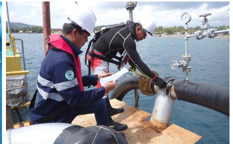
Above Water Dimensional Survey
