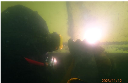
Installation of Formworks
