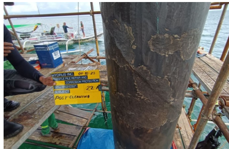
Post-cleaning of Corroded Steel Pipe Piles
