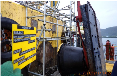
Dismantling of Existing Fender
