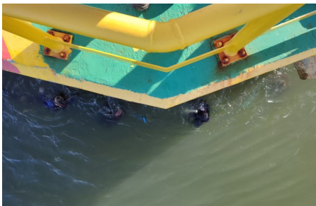
Removal of Marine Growth at Sidings and Soffit
