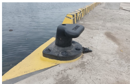
Installation of Marine Bollards and Marine Fenders
