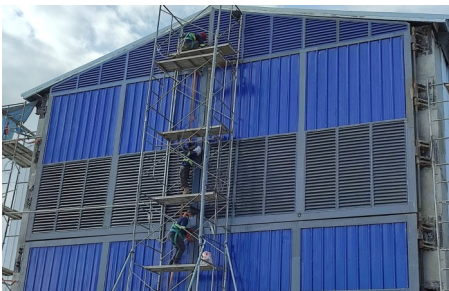
Installation of Hangar 2 Gate
