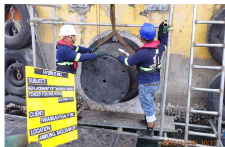
Installation of New Fender
