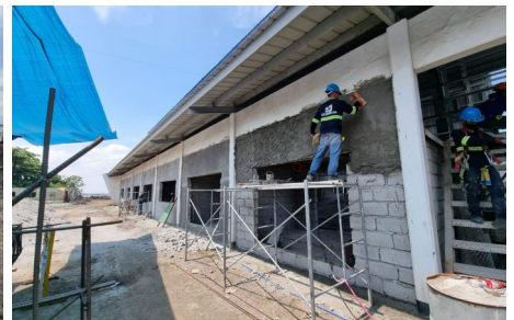
Rehabilitation of Hangar 2
