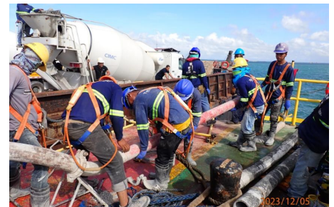
Concrete Placement
