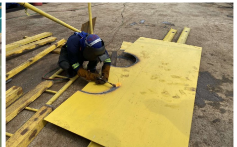
Fabrication of formworks
