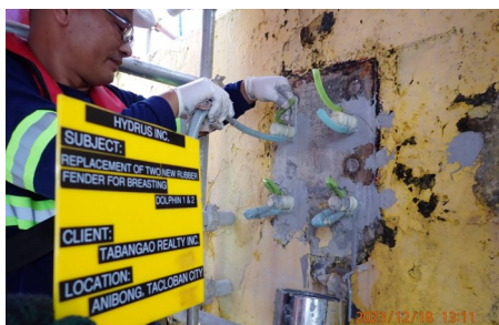
Grouting of New Bolts
